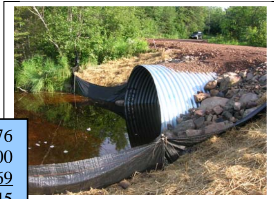
Access Road-Culvert Town of Anderson
